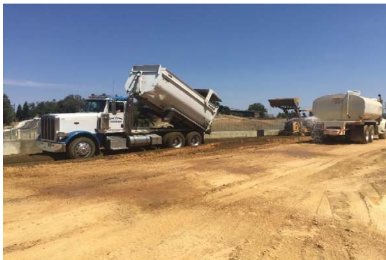
Pictured: structural backfill being placed behind the retaining wall
