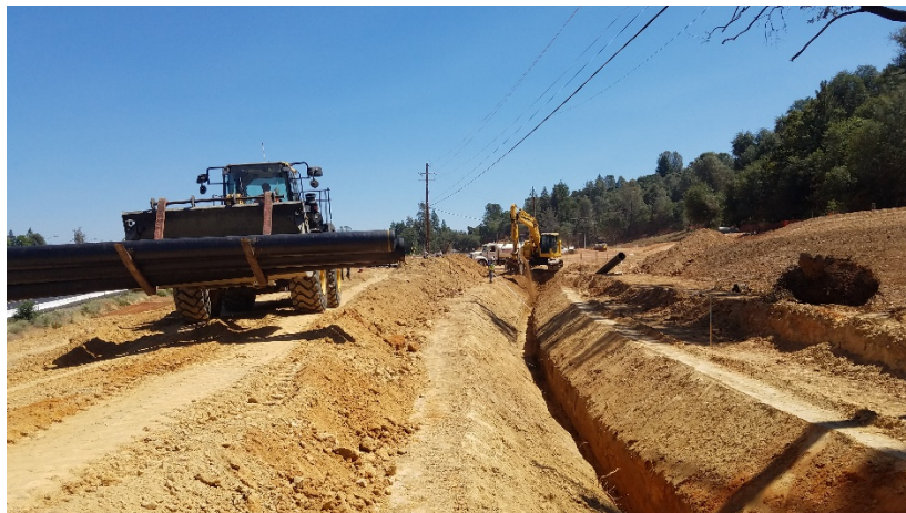
Pictured: Trenching for new 12" ductile iron water mainline
