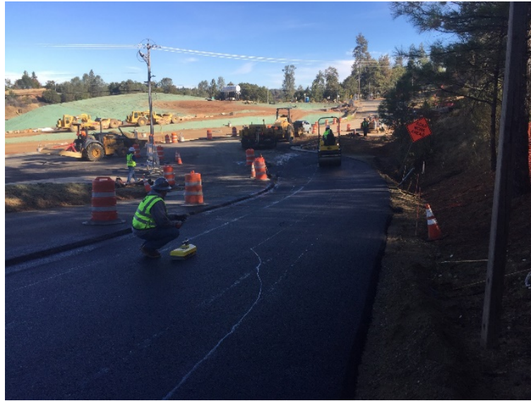
Pictured: Paving Eastern Half of County Jail Driveway
